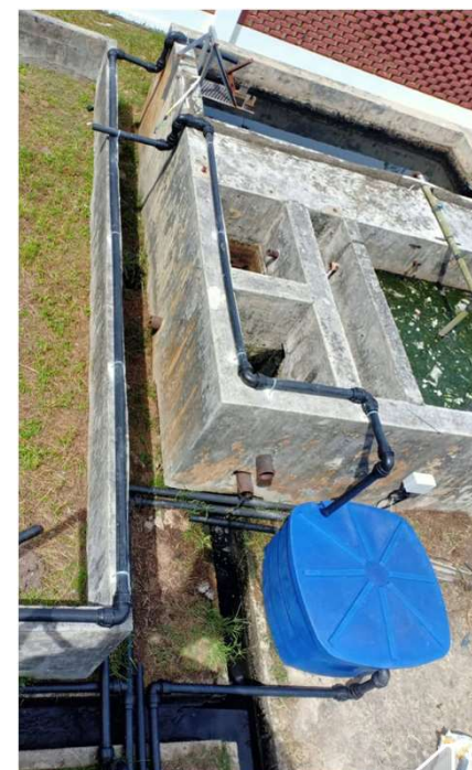
Pipe Work (8 days)
