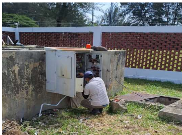
Electrical Construction Work (3 days)
