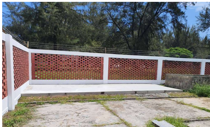
Foundation Construction (2 days)
