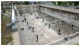
Installation of aerator
