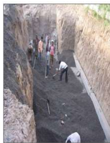
Filling with gravel size 4.5 to 12.5 mm
