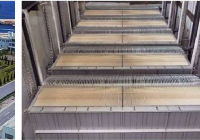
Submerged Membrane Unit (MBR)
