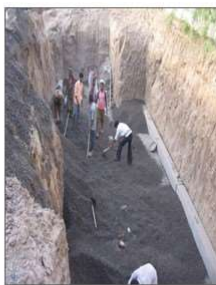
Filling with gravel size 4.5 to 12.5 mm
