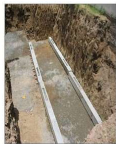
Filling with gravel size 4.5 to 12.5 mm
