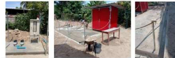
Blower and control panel Installation status Drainage ditch (for rainwater prevention)
