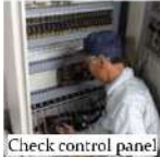
Check control panel
