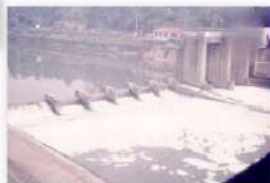
Chofu Weir, Tama River (Tokyo) in the 1970s
