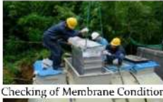
Checking of Membrane Condition
