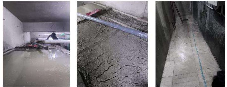
Case D Hotel : Improper grease trap design
