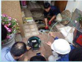
Inspecting the inside of the discharge pipe with an internal camera
