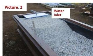
② Effluent inlet: The waterway was filled with pumice to a height of 28 cm. (upper part: Particle size 2~6mm, bottom part: Particle size 6~11mm)
