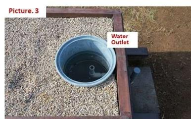
③ Water outlet: The water depth was set to 17cm. Runoff water passes through PVC pipes and flows into the biotope pond.
