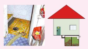
In many cases, decentralized wastewater treatment facilities such as septic tanks are installed under the floor of the houses. It is unsanitary when flooding occurs and requires to damage the floor for desludging. Decentralized wastewater treatment facilities should be installed at a certain distance by the outdoor wall of the houses.
