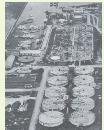
Picture 1 The first large scale night soil treatment plant (Sunamachi plant, capacity 3,600kℓ/day,1954) (6)
