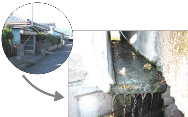
A road gully in tandoku-shori Johakasou installation area in 1970s (where whitish sludge was attached to)
