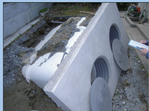
■ Tank pushed up to the surface by liquefaction
