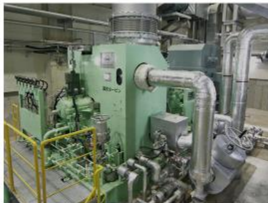
Steam turbine generator
