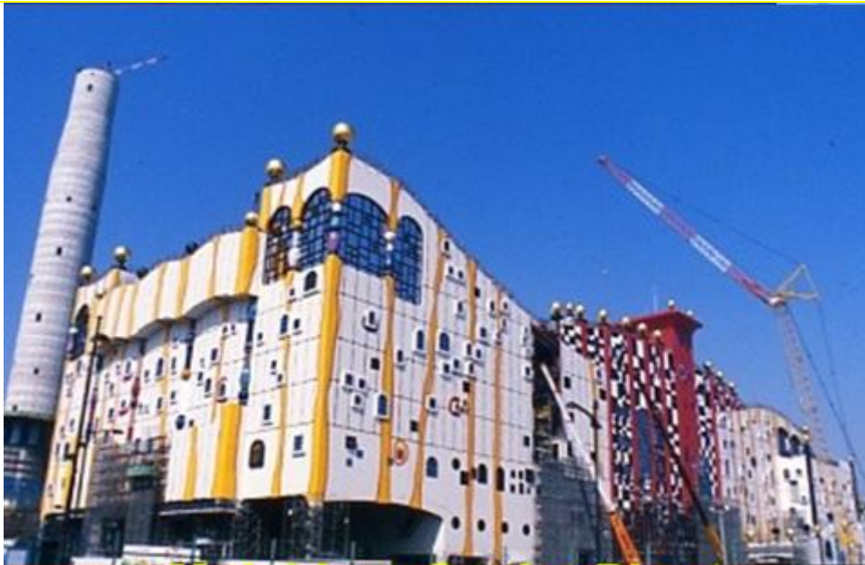
Maishima Osaka Plant under construction
