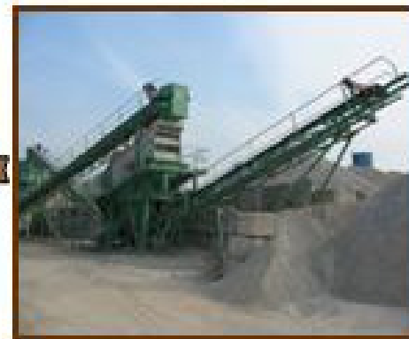
4) Further crushing and screening of RCA into various sizes
