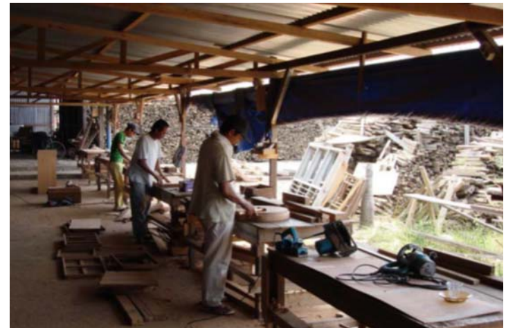
Repairment of window frames and doors
