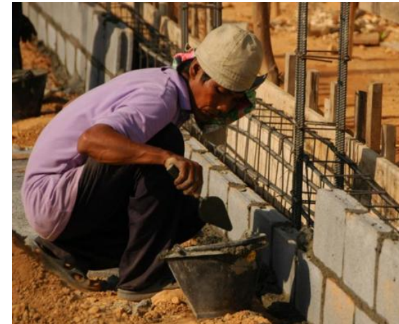
Construction activities after the tsunami
