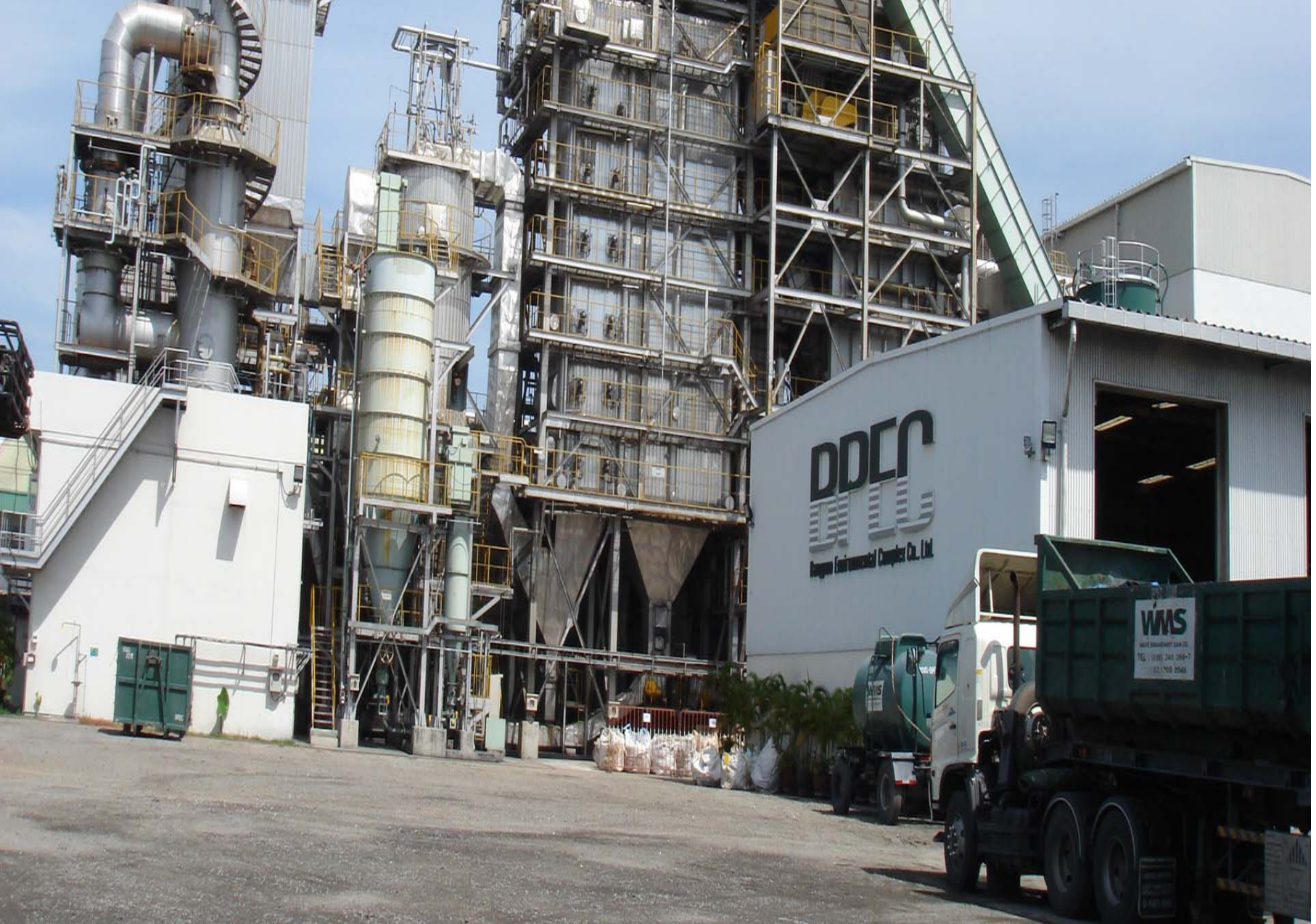
BPEC in Thailand Operates High Tech Incineration Plant
