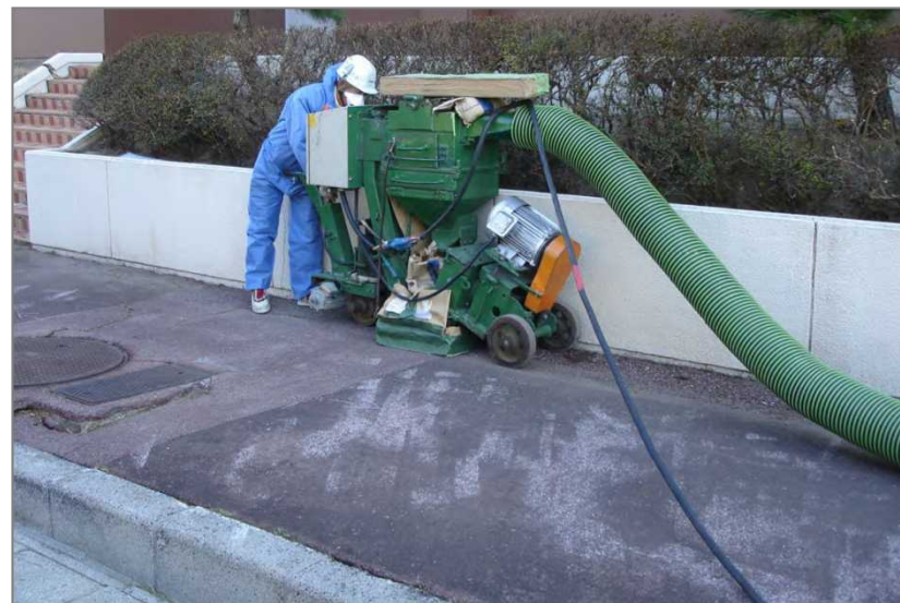
Shot-blast cleaning of sidewalk
