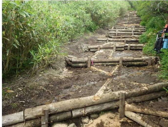
A photograph showing the same path after construction. The path is wider and more stable, with a wooden log barrier. The stream is now contained within a wooden structure. The path is surrounded by dense green vegetation. |
