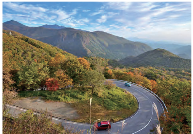
Second Iroha Slope for car traffic
