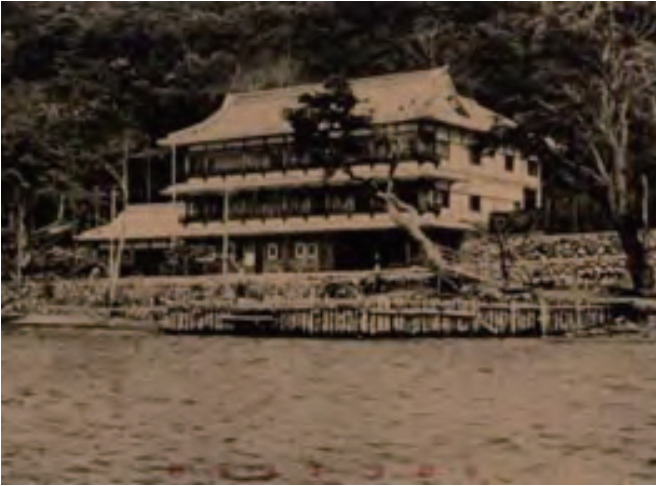
Former lakeside inn on Lake Chuzenji
