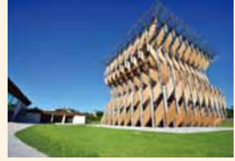
Kazenoha CLT pavilion
