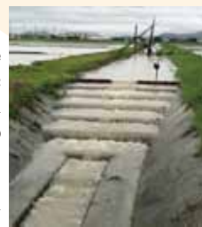
Fishway that allows fish to swim upstream
