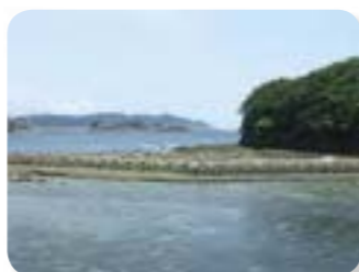
An existing breakwater levee
