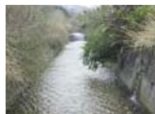
Channelized concrete canal in the wetlands
