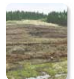
Contour log terraces for erosion control.
