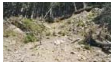
A slope failure site showing a lack of vegetation recovery in the Nishino-kawa River watershed.
