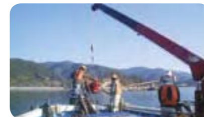
A small-sized crane and dredge pump
