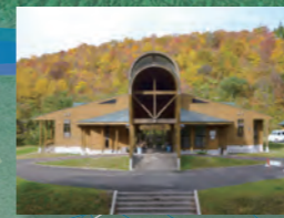
Shirakami-Promenade Kuromori-kan (Hall) This is a general information and rest area that is furnished with an exhibition hall and a break room. It is the starting point for a walkway from which visitors can see a part of the Kuromori (Black Forest). The forest has been protected in order to ensure water for paddy fields since some hundreds years ago.
