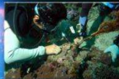
5) Underwater drilling with bolt attachments and plastic discs.
