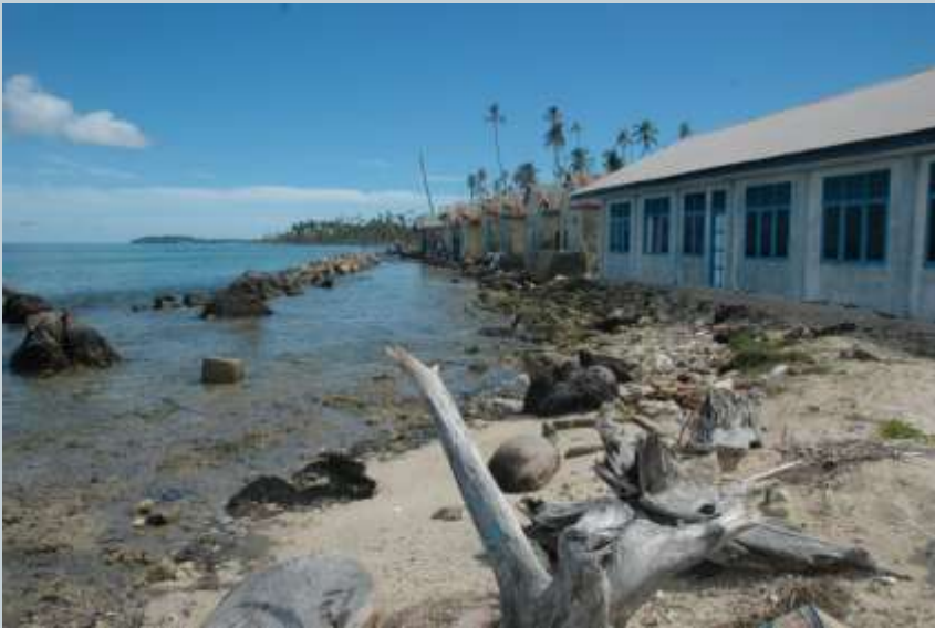
Coastal erosion at Balai Island of Banyak Islands
