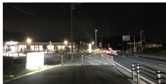
Power supply during blackout
