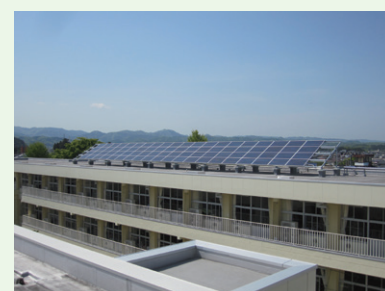
Solar panel installation subsidized by the government
