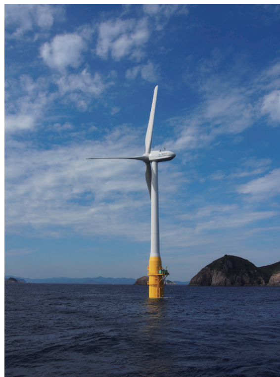
Floating offshore wind turbine demonstration project near Kabashima Island, Nagasaki
