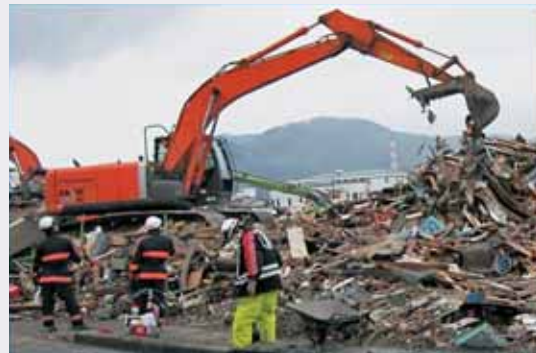
Removal of debris using heavy machinery
