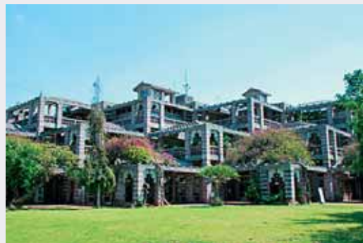
Nago City Hall, which was designed with the aim of not relying on large-scale air conditioning (Photograph provided by Nago City.)
