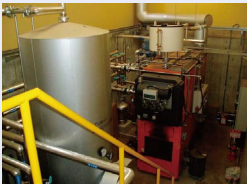
Photo3-3-1 Wood Biomass Boiler at Hadano City's Omotetanzawa Outdoor Activity Center
