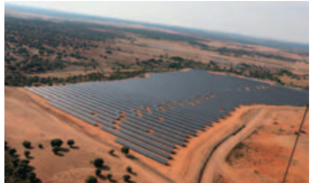
Planta Solar de Salamanca, a large scale PV power generation facilities in Salamanca, Spain (facility area: approximately 360,000m 2 ) (Photo: courtesy of KYOCERA Corporation)
