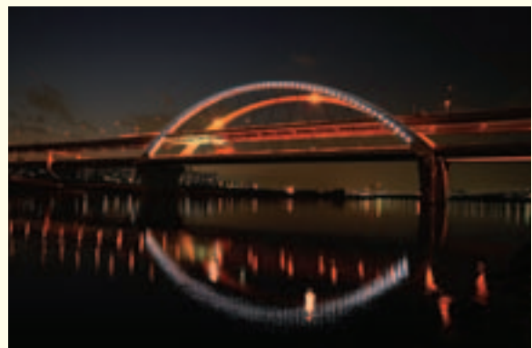
A bridge on an expressway lighted up using electricity from vehicle vibration
