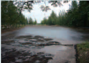
Anaerobic open lagoon on factory grounds (Ayutthaya Province, Thailand)
