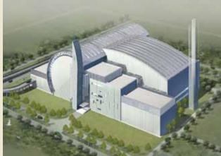
An electric generating facility with the capacity of 30,000 KW and steam condition of 4MPa and 400°C has been delivered to the incineration plant in Beijing, with capacity to handle 1,600t/day. Source:Takuma Co., Ltd.
