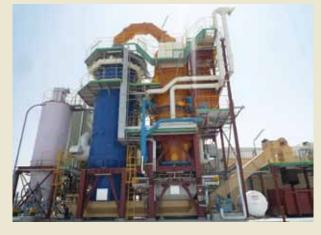
The medical waste incineration facility completed in Dobai is equipped with a vertical combustor that has the capacity to handle 19.2t/day and an air-purifying smoke and dust collection device for exhaust gas.
