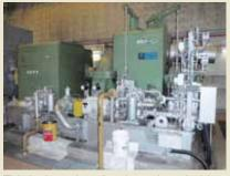
This incineration plant is equipped with a steam turbine generator that generates a maximum of 4,200kW, which is used in the plant. Excess electricity is sold to Tokyo Electric Power Company. The generator uses high-temperature water of 1Gcal/h, 130°C, with the maximum steam flow and pressure of 23.1t/h and 3.82MPa. (Shibuya Incineration Plant)
