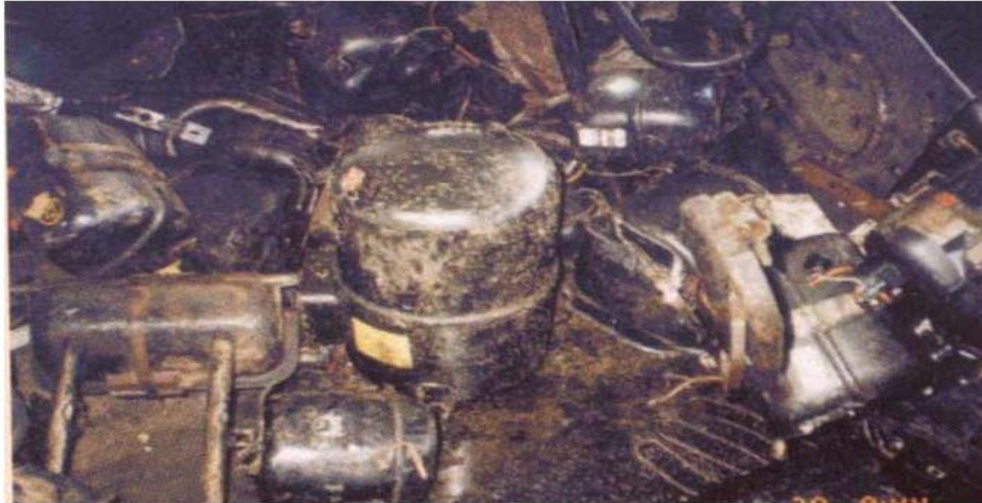
**Example of waste containing or contaminated with hazardous waste (PCBs waste) from Electrical utilities (transformers) which imported considered illegally (it stated in the import document as metal scrap).**
