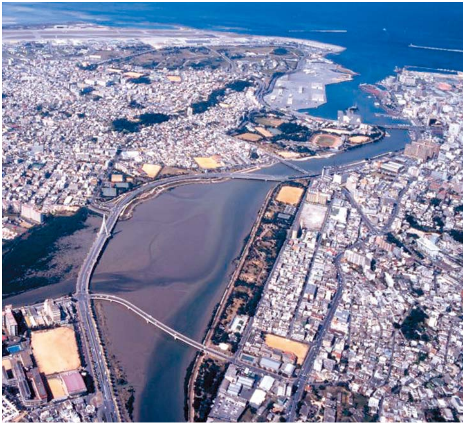
Aerial view of Manko from the east
