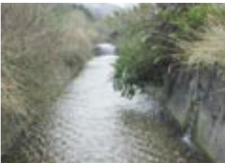
Channelized concrete canal in the wetlands
