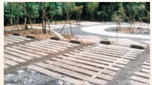
Timber-paved parking lot (Tanukiko Country Nature School, Fuji-Hakone-Izu National Park, Shizuoka).
