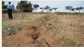
[ Rill erosion ] Ditch creation in areas of run-off concentration
