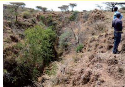
Over time, rills form larger gullies. Advanced gully erosion requires engineering work; it cannot be solved through the efforts of local people alone (Ethiopia).
