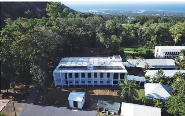
The PCCC located next to SPREP. Solar panels on the PCCC provide 20% of its electrical needs.
