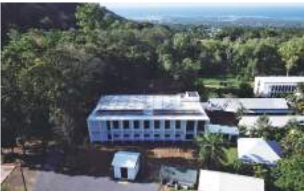
The PCCC located next to SPREP. Solar panels on the PCCC provide 20% of its electrical needs.
