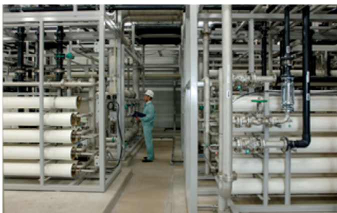
Reverse Osmosis Membrane Unit, the Core of Water Recycling
