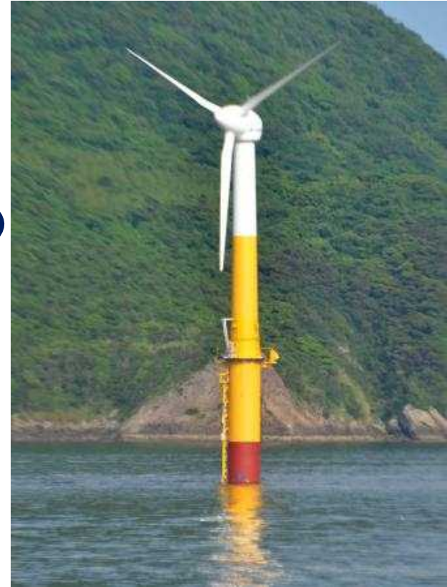
Offshore Wind Turbine installed by MOEJ
