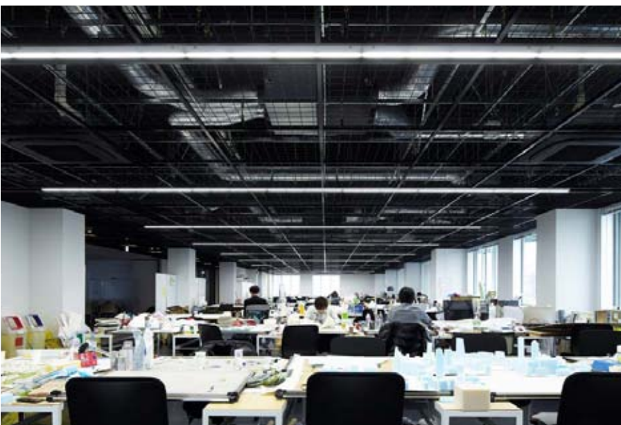
Drawing room. The mesh ceiling allows architecture students to see piping ductwork and other conduits that run above it. Slim LED lighting fixtures have been sandwiched between the mesh panels.
