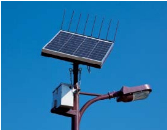
The combination of solar panels (80W) and lithium-ion batteries. The light source is white LED (10.8W).
