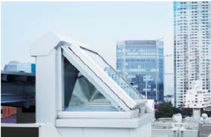
The skylight duct opening. Mirrors inside the ducts increase natural light reflection.
