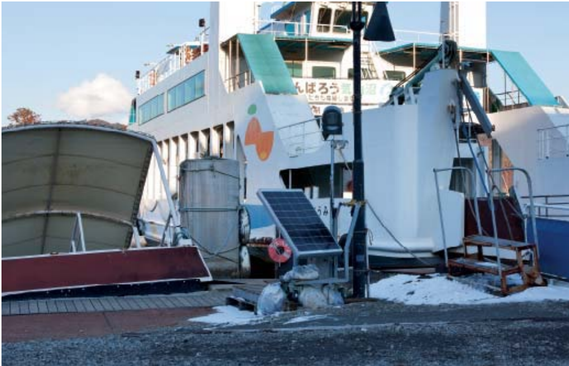
The portable solar panel installed at Oshima Kisen ferry terminal.
