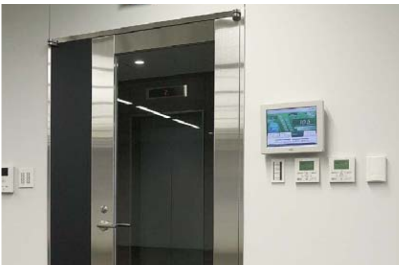
Energy-usage monitor. Placed in every office, these monitor screens detail current energy use to increase environmental awareness among users of the building.
