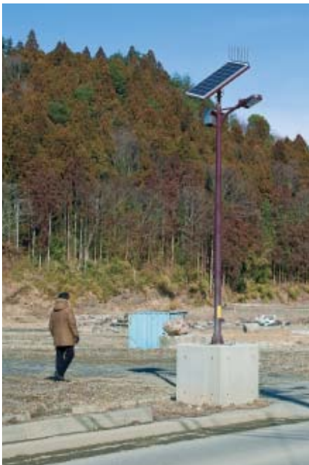
The light is 4m high excluding the base. The light base is usually buried under the ground, however, this large concrete base is exposed aboveground.
