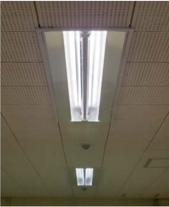
The light when switched on (stock image). Reflector panes concentrate the lighting and effectively project it towards the desk and wall surfaces, minimizing diffusion.
