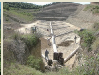
Semi-aerobic landfill facility under construction
