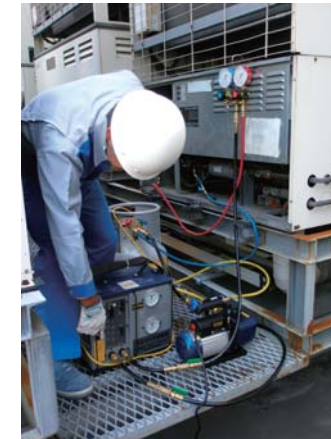
Recovery of refrigerant from super-market cold showcase Source: Refrigerants Recycling Promotion and Technology Center, Japan
