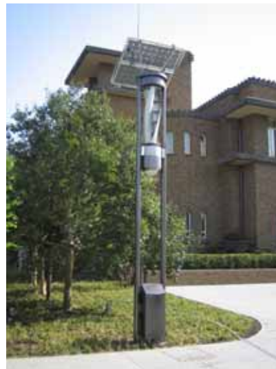
➤ Wind Power Generation
