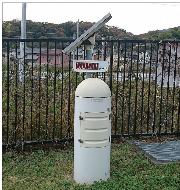
Actual measuring instrument (radiation monitoring post)
