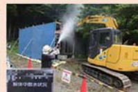
Demolition of a damaged house, etc.
