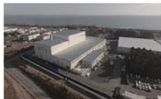
Temporary Incineration Facility in Okuma Town (December 2017)
