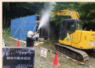
Demolition of a damaged house, etc.
